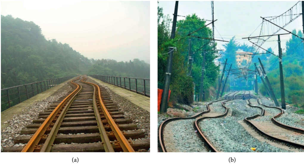
FIGURE 1: The earthquake paralyzed the railway system.
