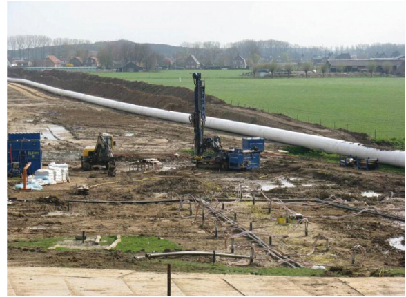
FIGURE 14: Field test of MICP foundation reinforcement [113].
