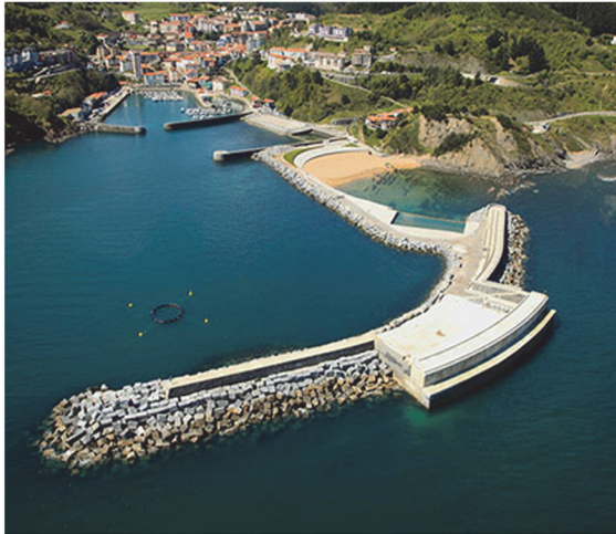
FIGURE 1: The OWC power plant of Mutriku.
