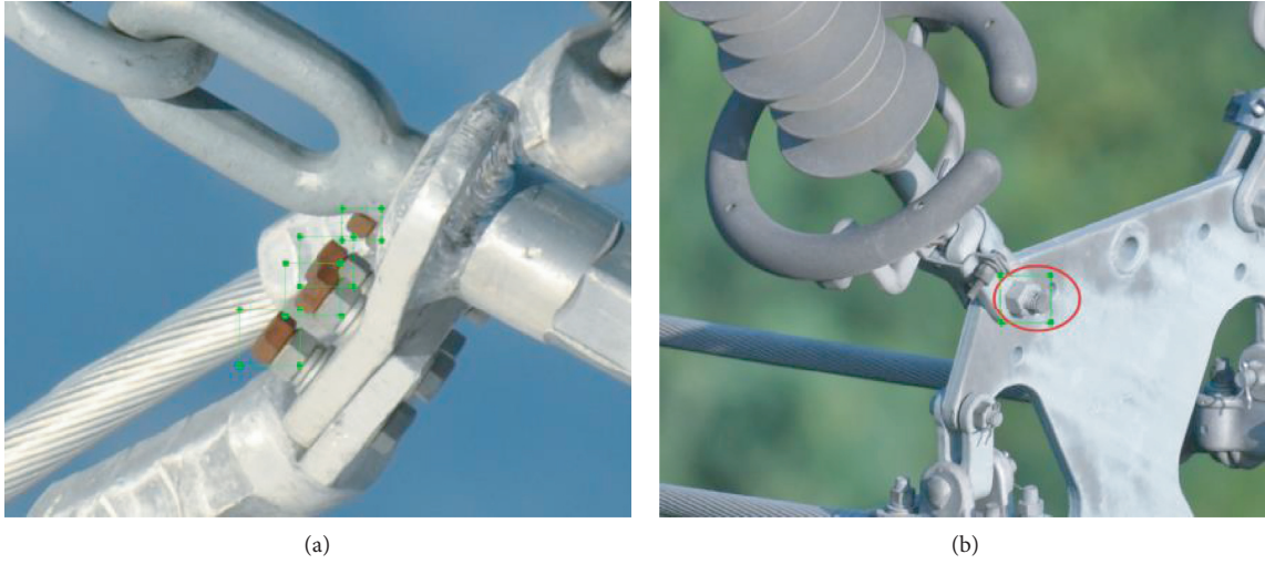
FIGURE 1: Pin-level defect. (a) Rusted-on nut. (b) Lack of locking pin.
