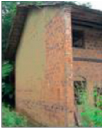
FIGURE 2: Mixed masonry method.
