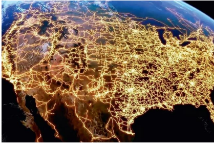
FIGURE 9: A huge power grid system with isolated grids connected by long-distance transmission lines.
