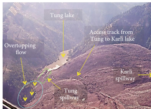
FIGURE 7: (a) Cross-section of the deepest spillway cut along the landslide dam portion blocking Tung lake; (b) photograph of Tung lake overflowing newly excavated spillway (February 12, 2006).
