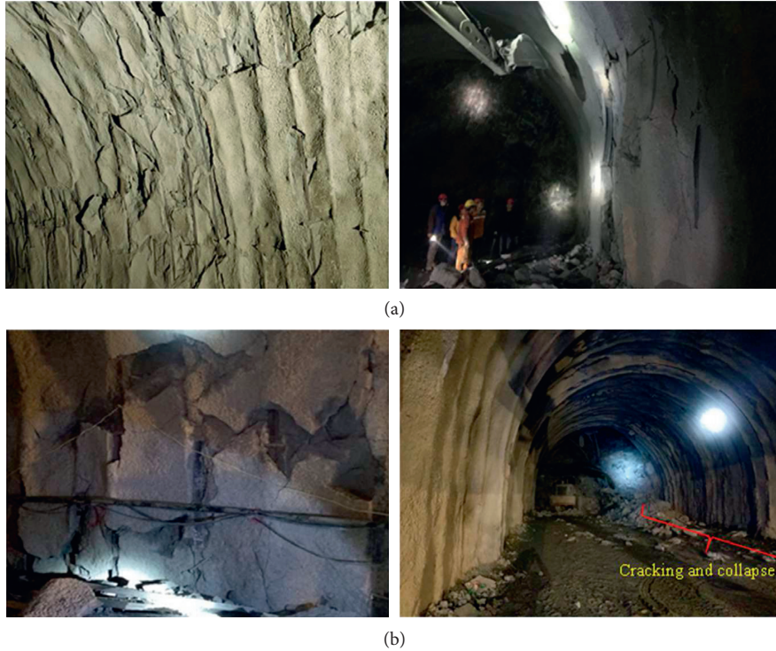
FIGURE 16: The lining crack before and after rockburst: (a) before the rockburst; and (b) after the rockburst.
