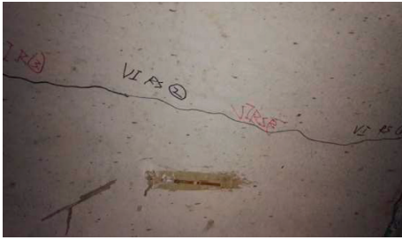
FIGURE 18: Destruction diagram of the right spandrel at the entrance of the tunnel.
