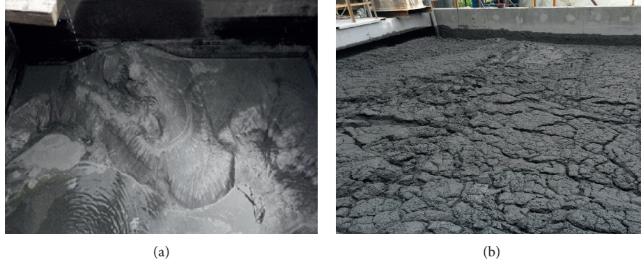
FIGURE 1: Muddy foams on the liquid surface in XTM: (a) initial operation; (b) after 7 days.
