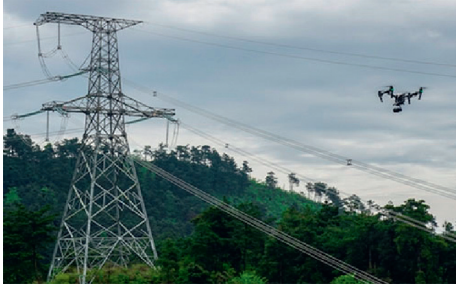
FIGURE 1: UAV-based autonomous transmission line inspection.
