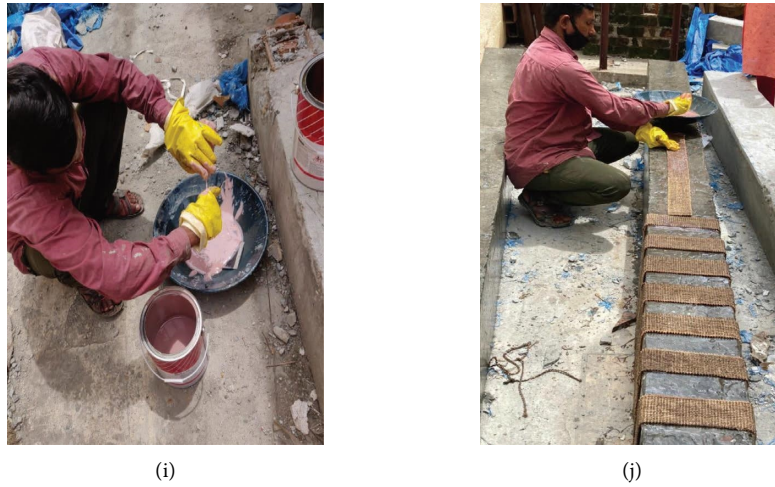
FIGURE 5: Experimental procedure followed (a) reinforcement, (b) sheathing pipe positioning, (c) reinforcement for installation, (d) positioned in shuttering, (e) concrete filling and compaction, (f) curing, (g) post tensioning, (h) filler application, (i) resin preparation, and (j) retrofitting with FRP.
