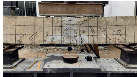
FIGURE 4: Failure state of the test beam.
