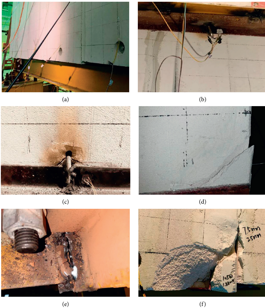
FIGURE 14: Test results of FW1. (a) Obvious dislocation between panels. (b) Angle steel weld fractured. (c) Extended cracks at bolt holes. (d) The broken phenomenon of the panel angle. (e) Weld fractured. (f) Large areas of damage in each panel corner.
