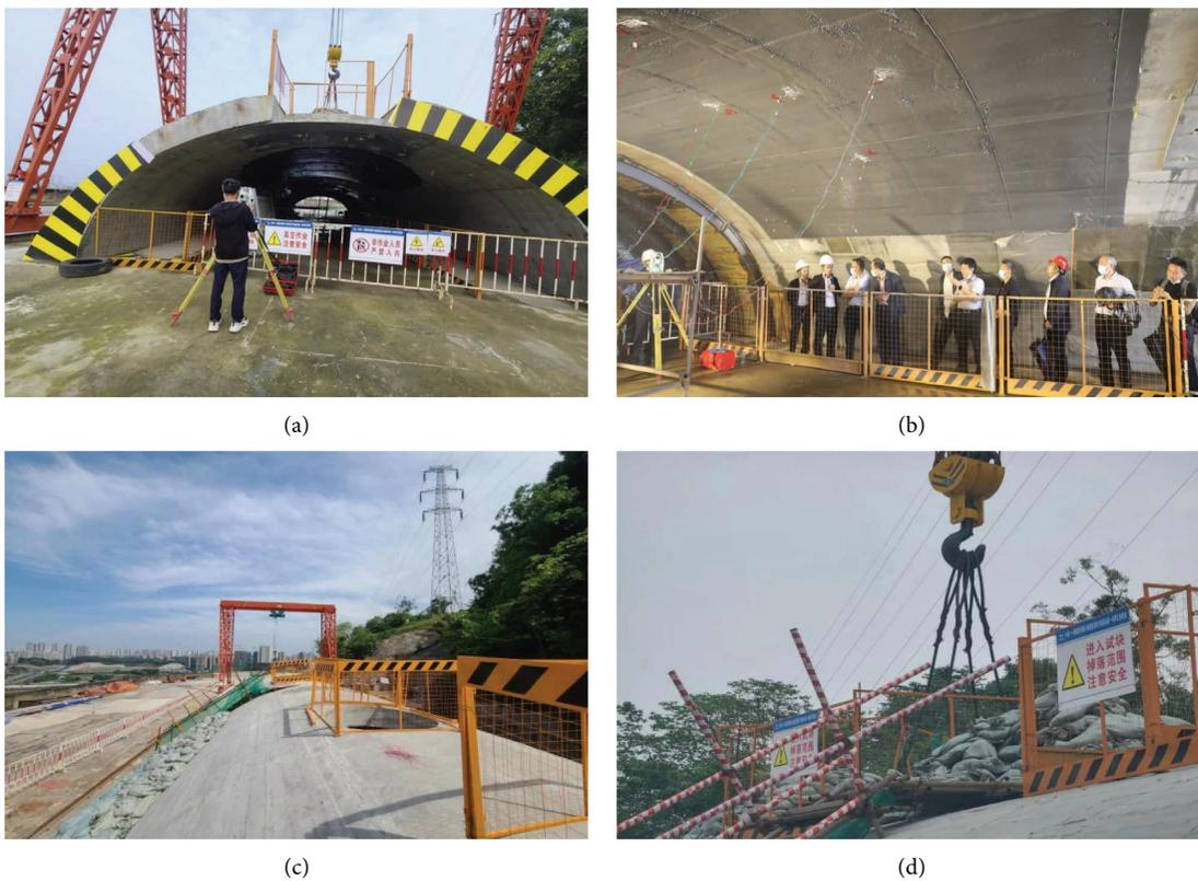
FIGURE 12: Construction safety control. (a) Tunnel model entrance isolation. (b) Tunnel model internal isolation. (c) The tunnel model was fully enclosed and isolated. (d) Warning signs around the vault test block.
