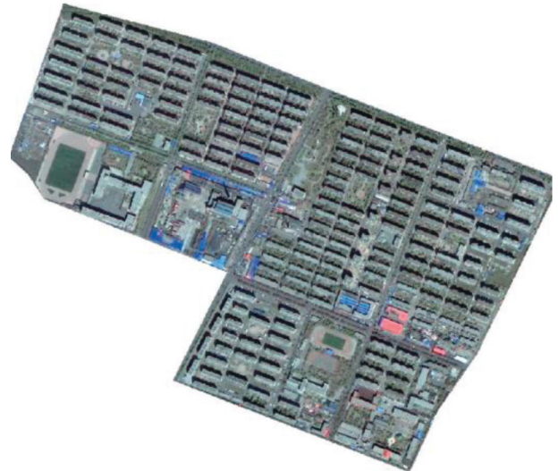
FIGURE 7: Geometry spatial composition and color planning of public buildings in smart cities.
