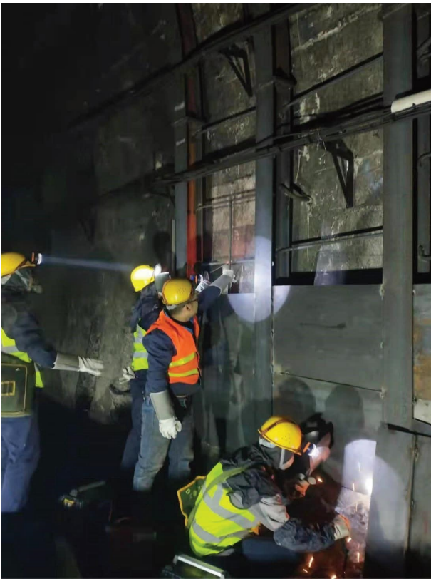
FIGURE 19: Installation site of connecting reinforcement and steel plate.
