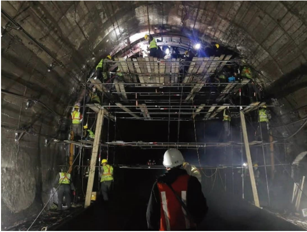
FIGURE 18: Installation site of steel arch.
