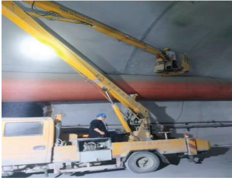
FIGURE 12: Lining construction quality inspection site.
