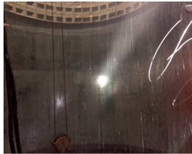
FIGURE 4: HPC shaft lining after form stripping.
