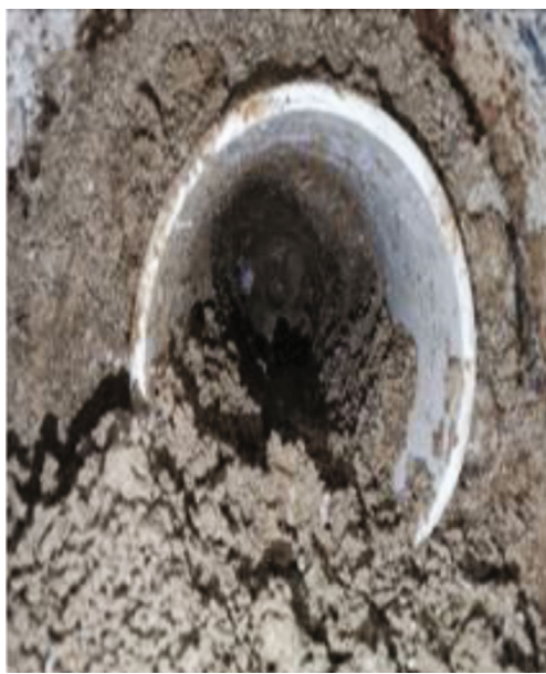
(g) Seventh excavation
