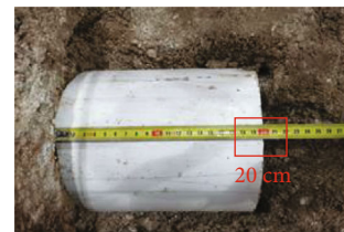
FIGURE 10: The embedment of the PVC pipe.
