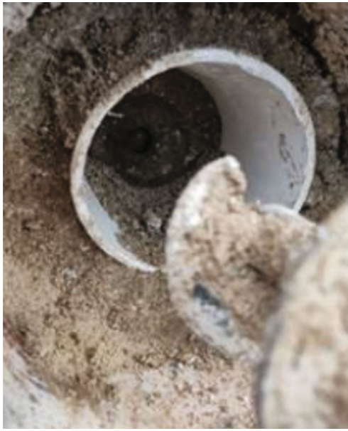
(a) First excavation
