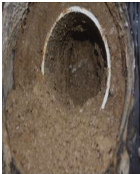
(h) Eighth excavation
