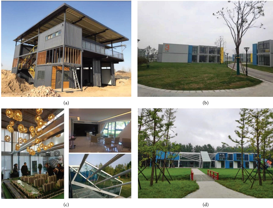
FIGURE 9: Photo of pilot projects. (a) Container modular fire station under construction. (b) Photo of “Xiangyu” residence in Yangzhou software park. (c) Indoor photo of the container pilot project. (d) Photo of Yangzhou Suburb park maker center.
