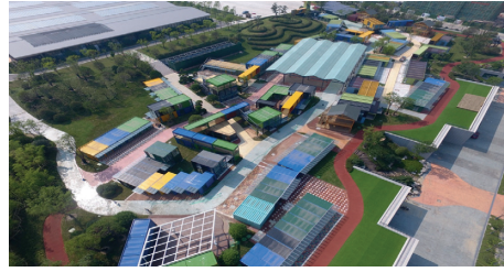
FIGURE 1: Pilot project-real aerial photo of Huaduhui Commercial Street.
