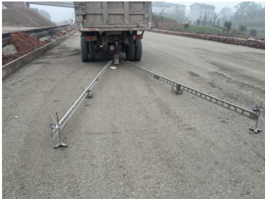
FIGURE 1: Field test of the bearing plate.
