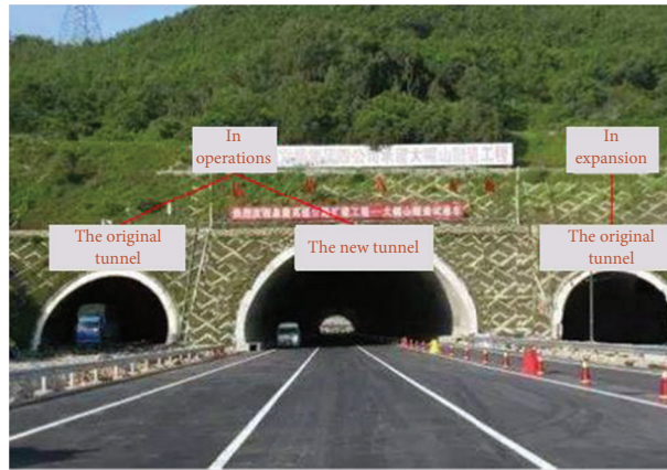
FIGURE 2: Illustration of reconstruction and expansion of tunnel.
