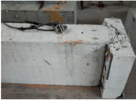
FIGURE 15: Failure diagram of precast beam.
