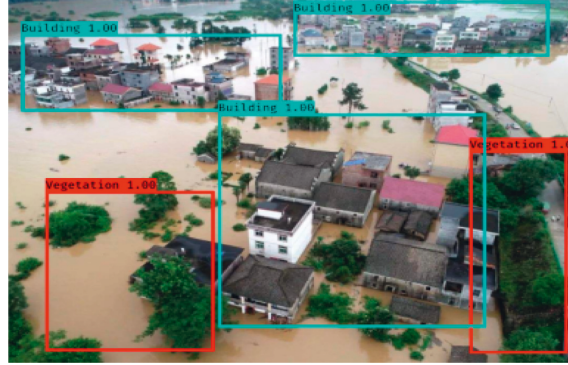
FIGURE 12: Example of flooded building area estimation.
