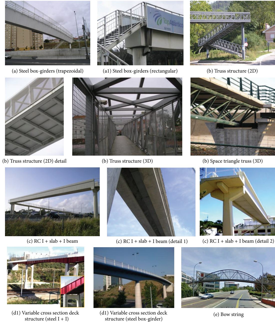
FIGURE 3: Main typologies of footbridges in Portugal.
