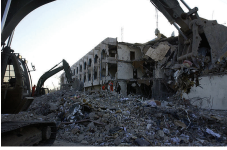
FIGURE 1: Destroyed reinforced concrete building by blast load [15].
