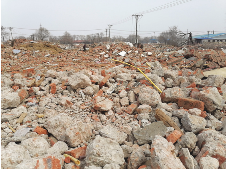
FIGURE 1: Appearance of construction waste.
