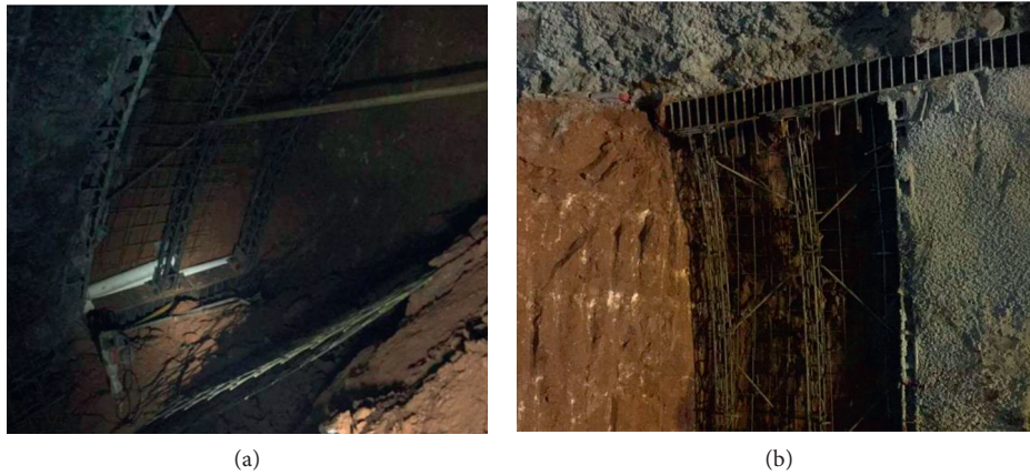
FIGURE 10: SRLD after construction. (a) Upper step. (b) Middle step.
