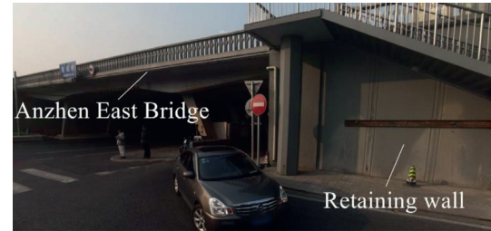
FIGURE 1: Image of Anzhen East Bridge and the retaining walls.
