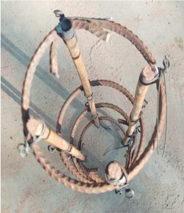
FIGURE 7: Reinforcements used in column casting.
