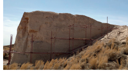
FIGURE 1: The reinforced site wall.
