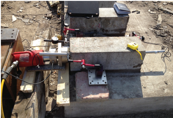
FIGURE 7: Setup of the scale horizontal push plate test.
