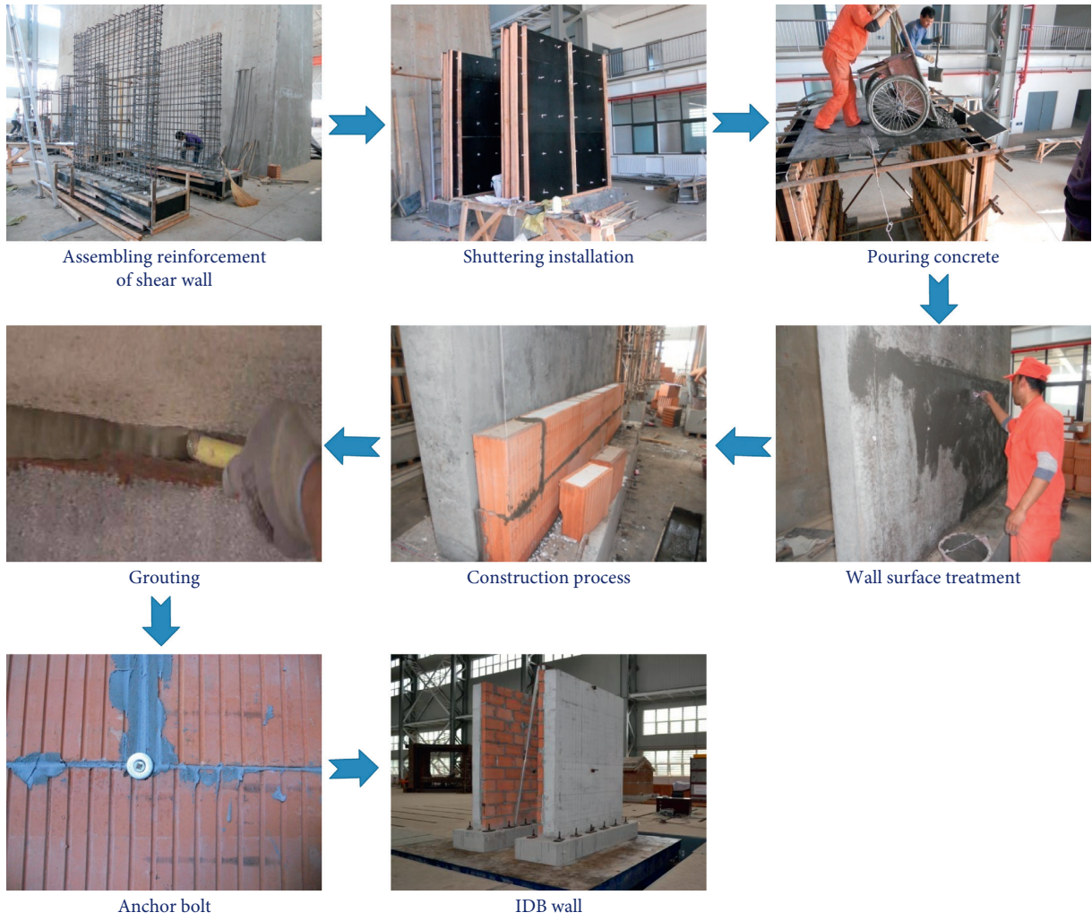
FIGURE 4: Construction process of specimens.
