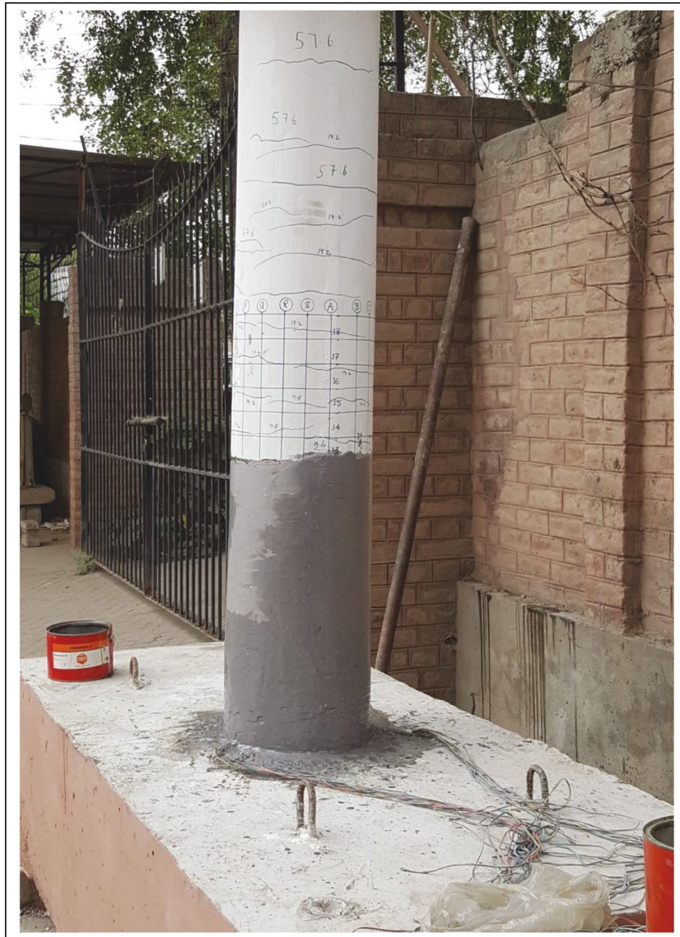
FIGURE 5: Grinded and prepared surface of pier for CFRP application.
