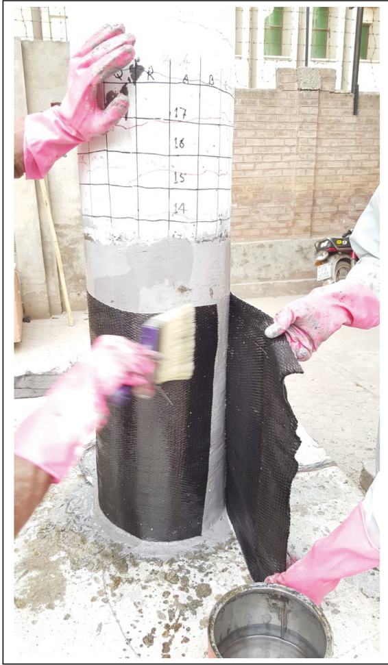
FIGURE 6: Application of CFRP (HEX-103-C) to pier.
