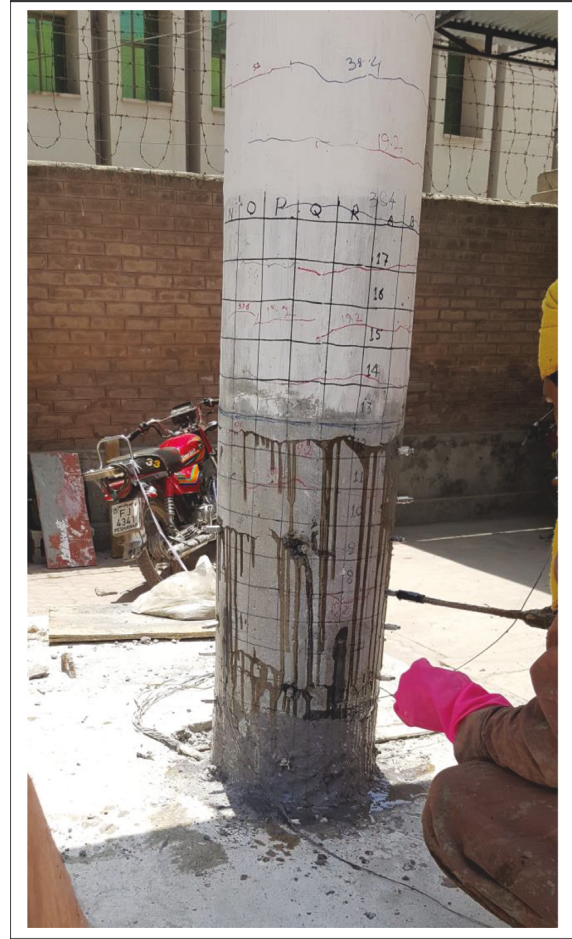
FIGURE 4: Outer repair works with cementitious mix after filling of cracks.
