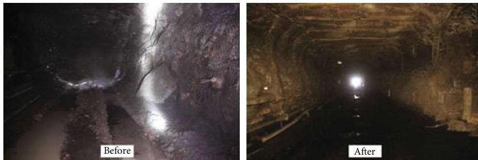
FIGURE 19: Effect picture of entry staying along goaf before and after roof failure pressure relief.
