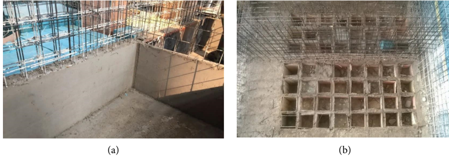
FIGURE 3: Construction of the concrete model. (a) Shear wall; (b) spent-fuel pool.
