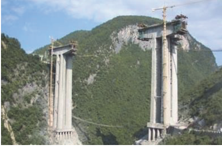
FIGURE 1: Yesanhe Super Large Bridge in construction.
