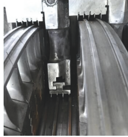
FIGURE 1: High pressure stage of steam turbine in power plant.
