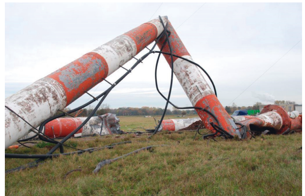
FIGURE 8: Guyed mast debris section partly penetrated into the ground.
