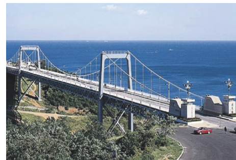
FIGURE 5: Dalian Northern Suspension Bridge.
