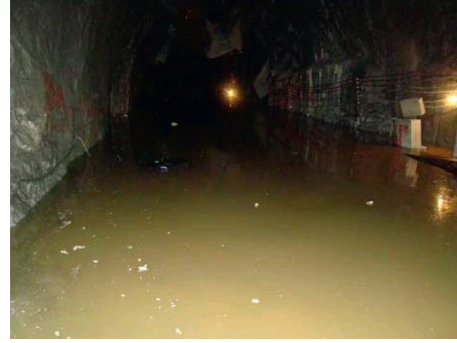
FIGURE 5: The picture of water discharge of the roadway in 8 h after water inrush.
