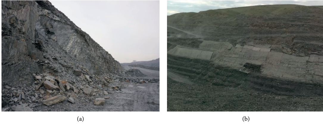
FIGURE 2: Instability failure of open-pit mine in current situation. (a) Collapse in mining area. (b) Re-instability of reinforced area.
