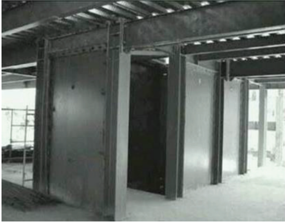
FIGURE 1: Executing steel shear wall.
