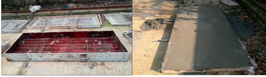
FIGURE 4: Concrete slab processing.
