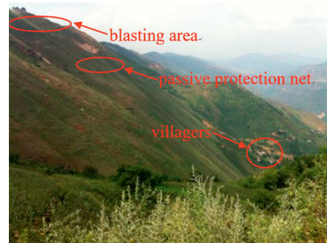
FIGURE 1: Surrounding environment of the blasting area.
