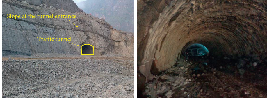
FIGURE 2: No. 2 traffic tunnel at the Baihetan hydropower station.
