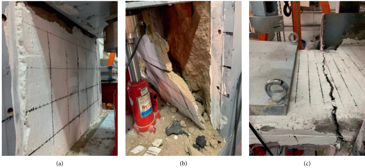
FIGURE 4: Roof and face failures of the physical models under dynamic roof loading: (a) face buckling; (b) face fall; (c) roof fall.
