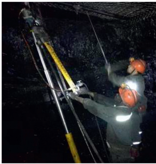
Drilling process of roofbolter
