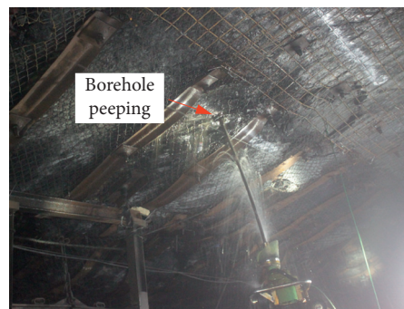
FIGURE 11: Illustration of borehole peeping construction.
