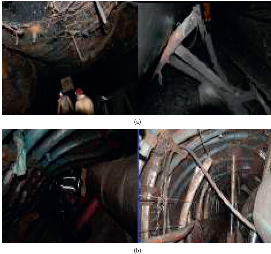
FIGURE 1: Typical mine earthquake disaster results caused by thick and hard rock strata movements. (a) Site image of a “2.28” mine earthquake disaster in the Gucheng Coal Mine of Shandong Province. (b) Site image of an “11.3” mine earthquake disaster in the Qianqiu coal mine of Henan Province.
