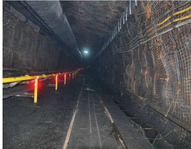
FIGURE 20: Stable section of the roadway.
