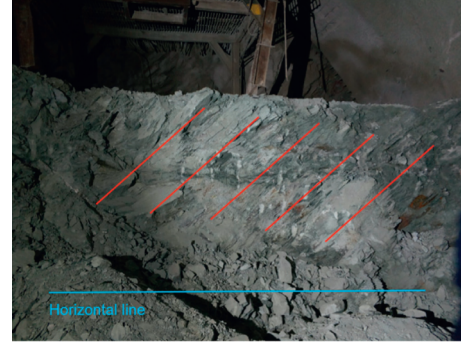
FIGURE 2: Bedding structure of surrounding rock of Xiangli Expressway Tunnel in Yunnan Province.
