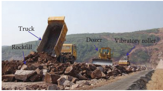
FIGURE 1: Vibratory roller compaction of field rockfills.
