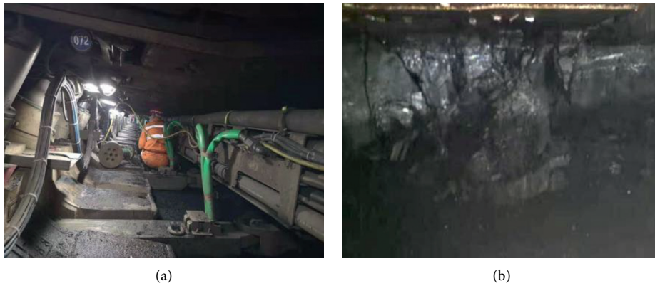
FIGURE 3: Support crushing and coal wall collapse in the 22306 working face, Shigetai mine.
