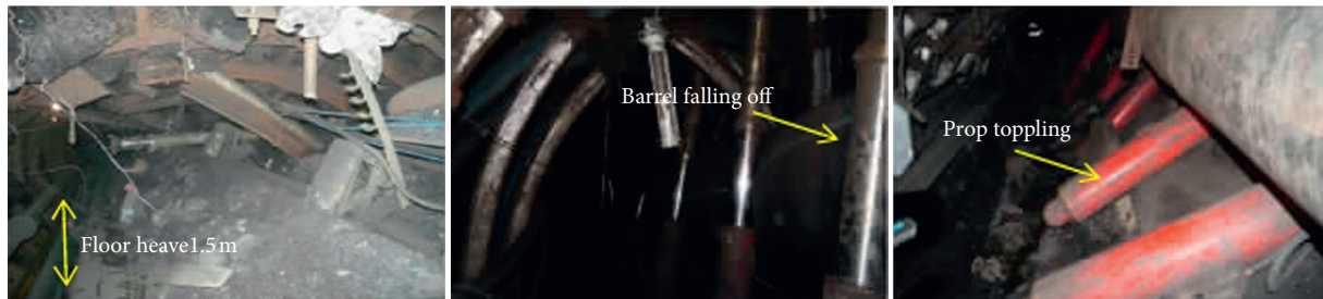
FIGURE 7: Scene photos of roadway rock burst accident in Qianqiu mine.
