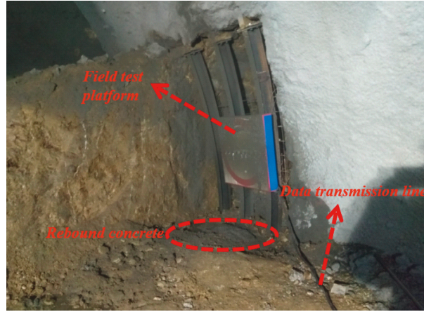
FIGURE 1: Field test platform.
