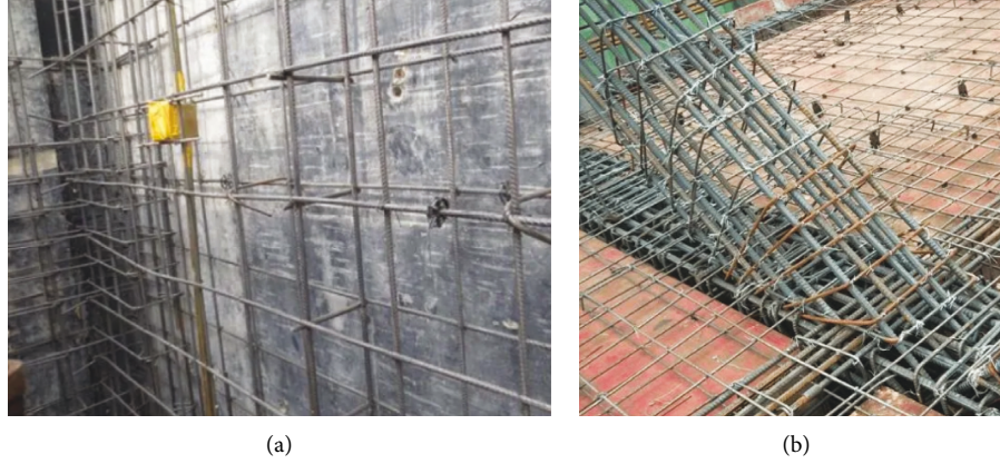
FIGURE 4: Actual reinforcement diagram of shear wall and beam members. (a) Actual reinforcement drawing of the shear wall. (b) Actual reinforcement drawing of the beam member.
