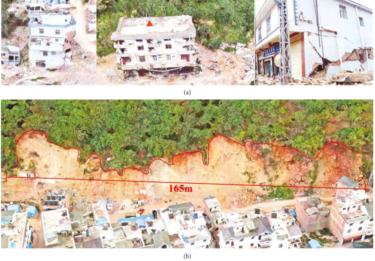
FIGURE 7: Typical seismic damage phenomenon in Longtou Village in Ludain Ms 6.5 earthquake. (a) Damaged buildings. (b) Landslides.
